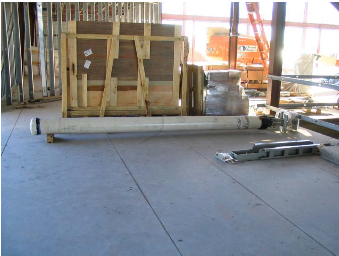
Visitor elevator equipment has arrived
