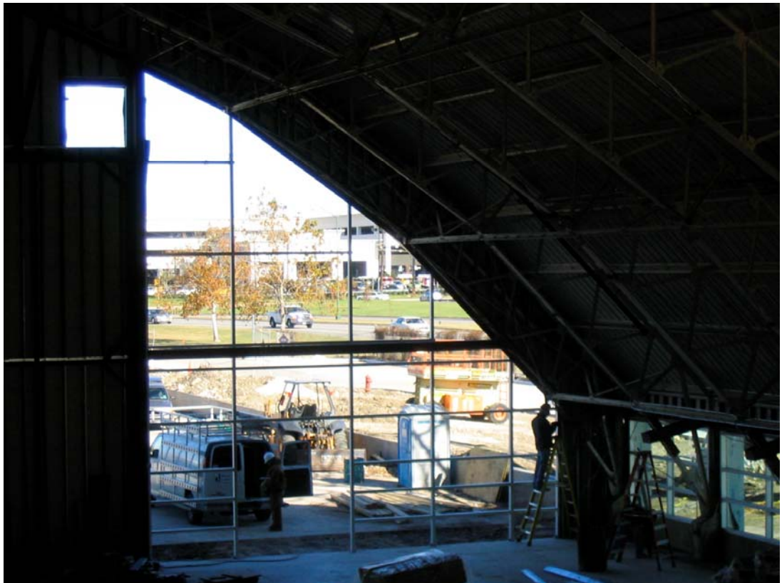
Window framing in old hangar
