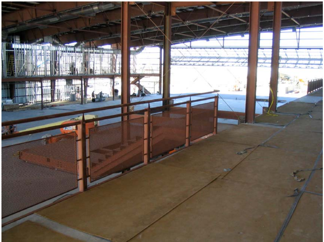
2nd floor railing being installed
