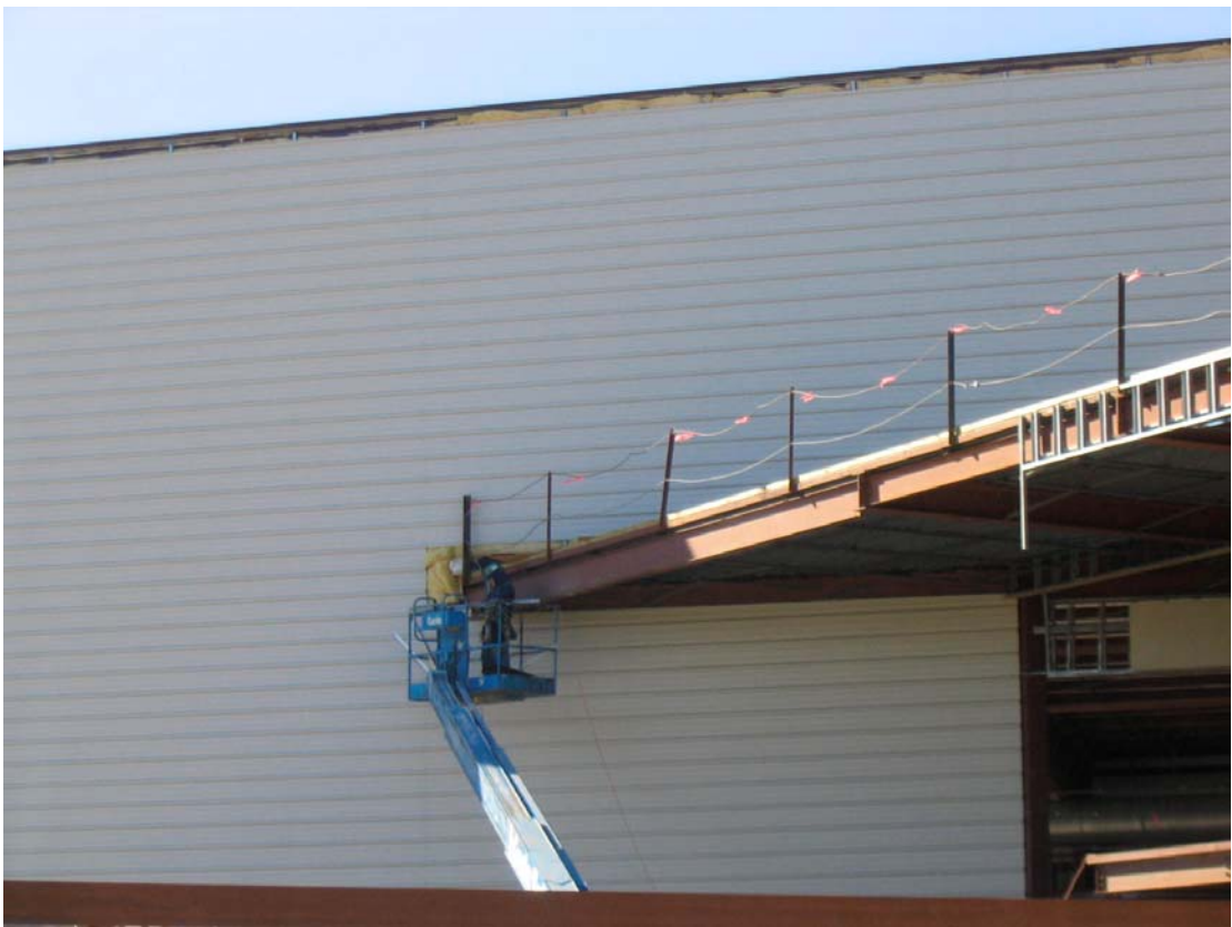
Main hangar siding work continues
