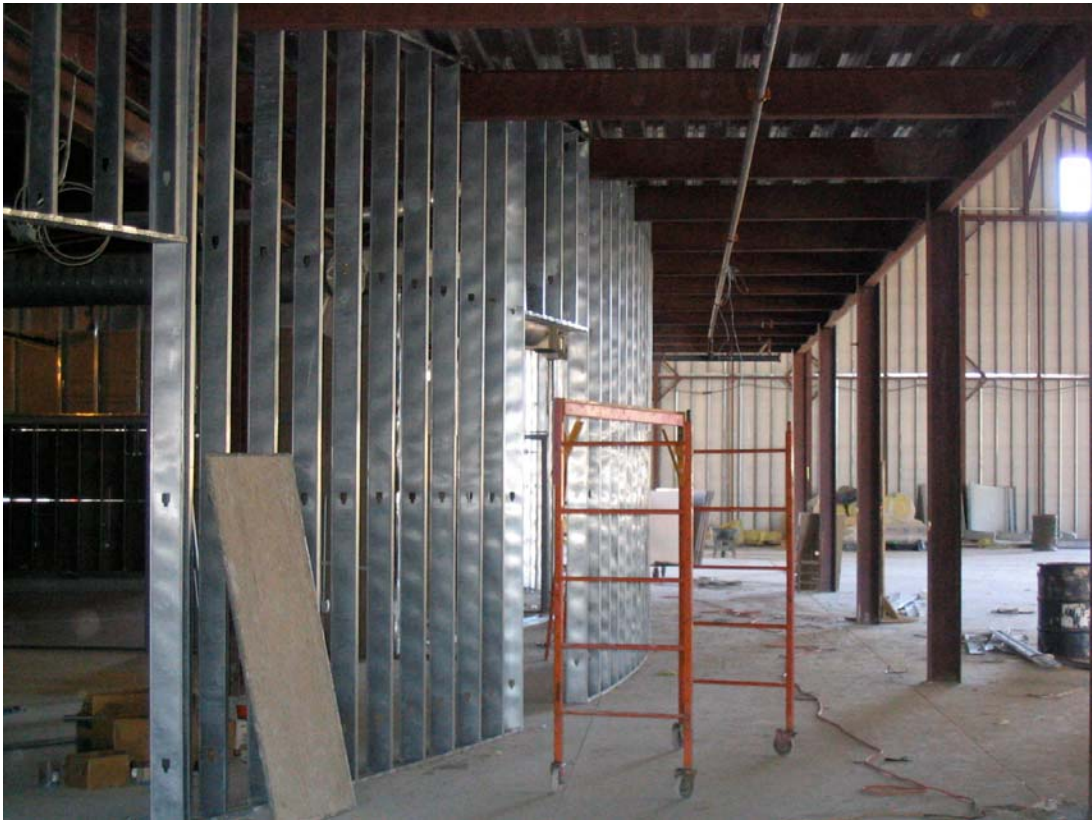
Now that concrete pours finished, 1st floor walls going up
