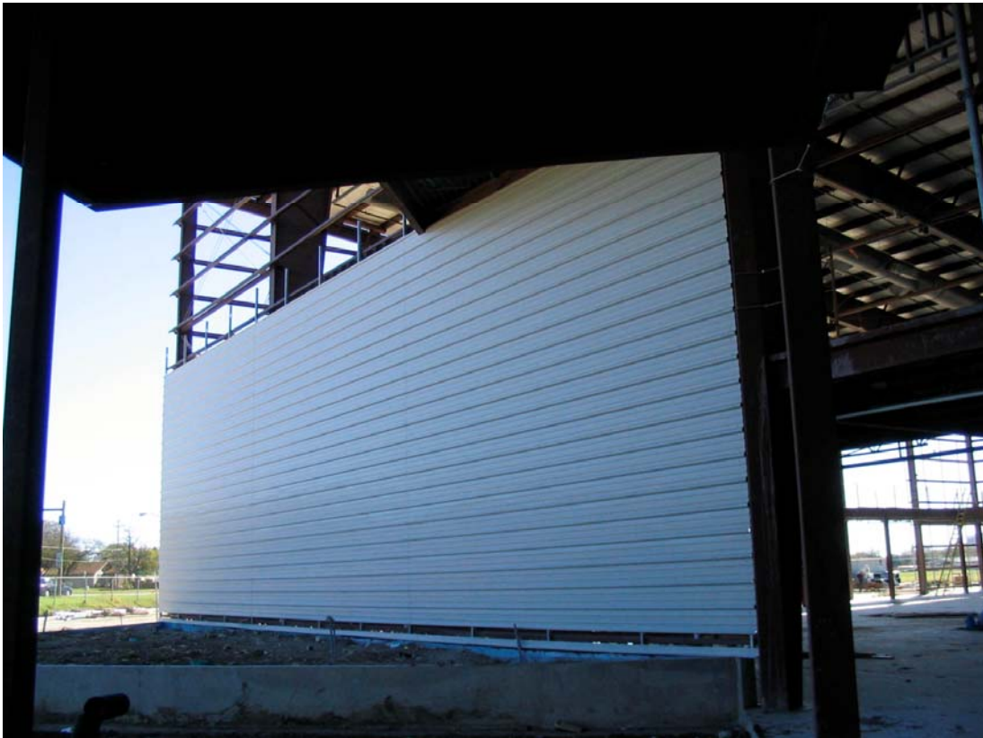
Main hangar siding finally going up
