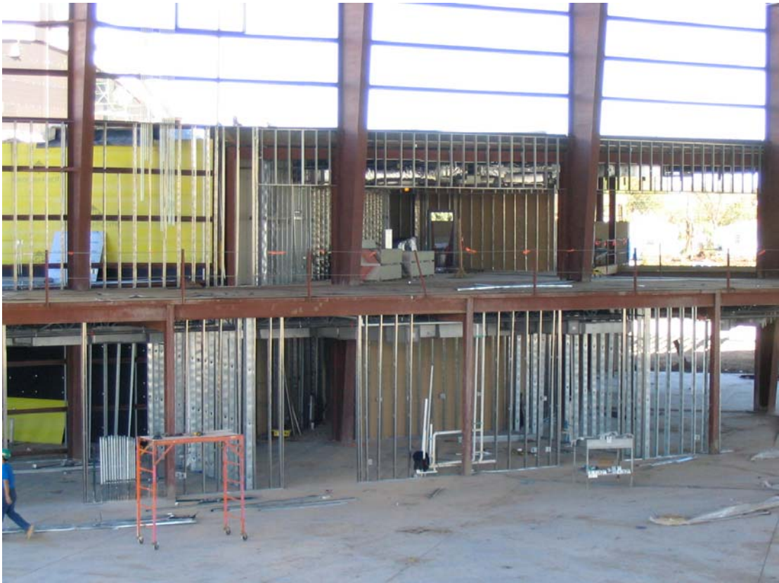
Interior wall work continues
