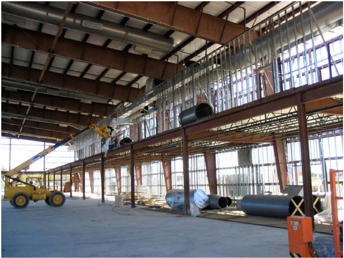
Offices on mezzanine in new hangar going up
