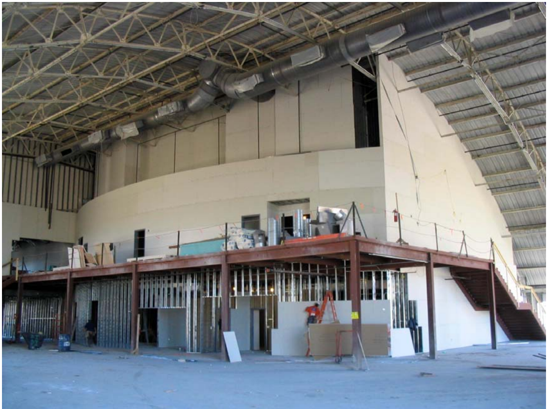
Auditorium and classrooms below taking shape
