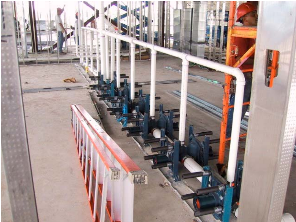
Upstairs plumbing lines up
