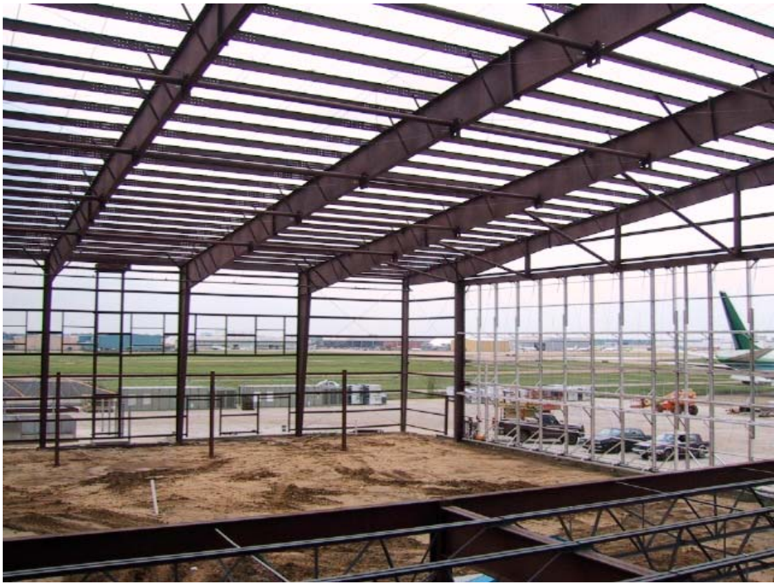
View of main hangar from mezzanine
