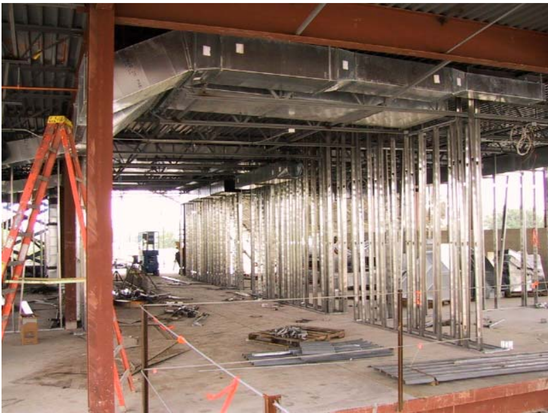
2nd floor wall studs going up
