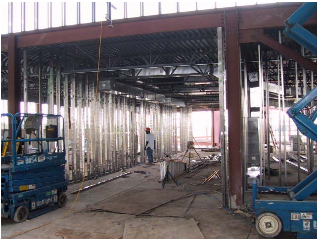
2nd floor walls going up - shot 2
