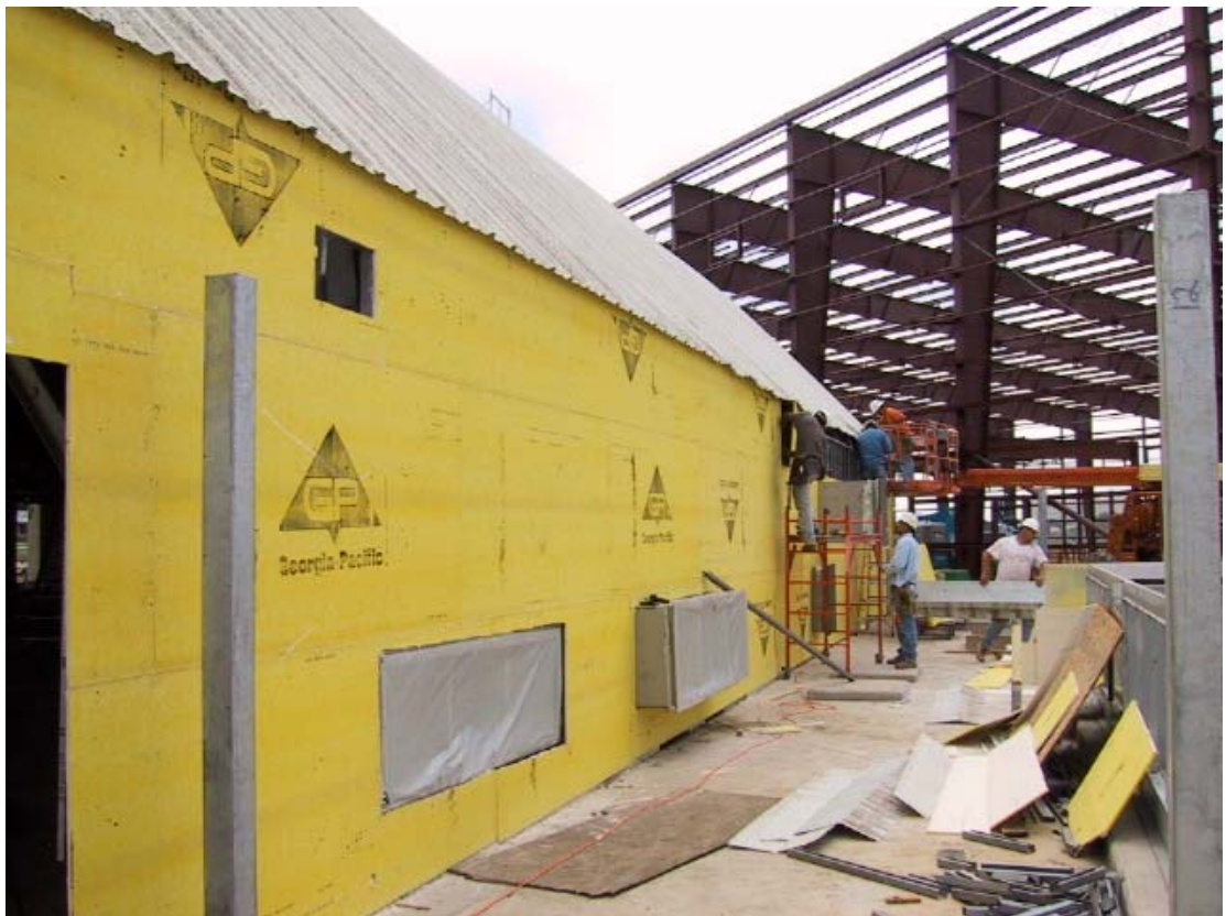
Outside wall insulation going up
