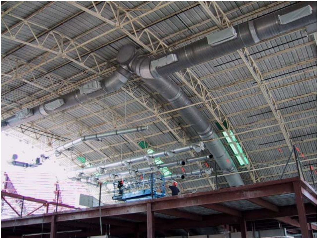
2 nd floor HVAC continues to grow
