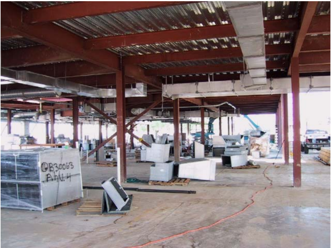
1 st floor HVAC ducting work continues
