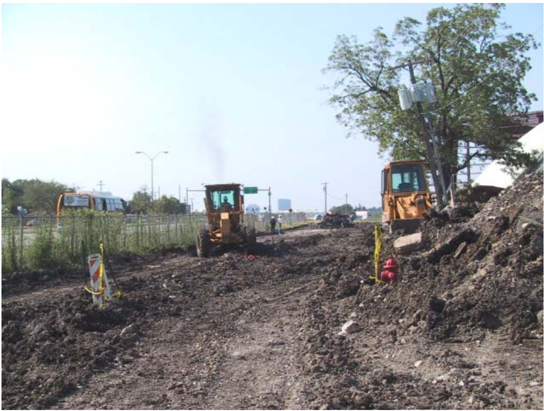
New parking lot work continues
