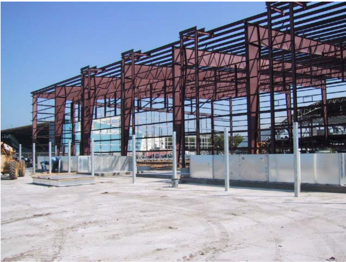
Pad and enclosure for outside air HVAC equipment being installed
