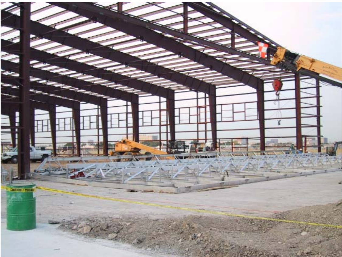
New hangar bi-fold door being installed - 110' x 22'
