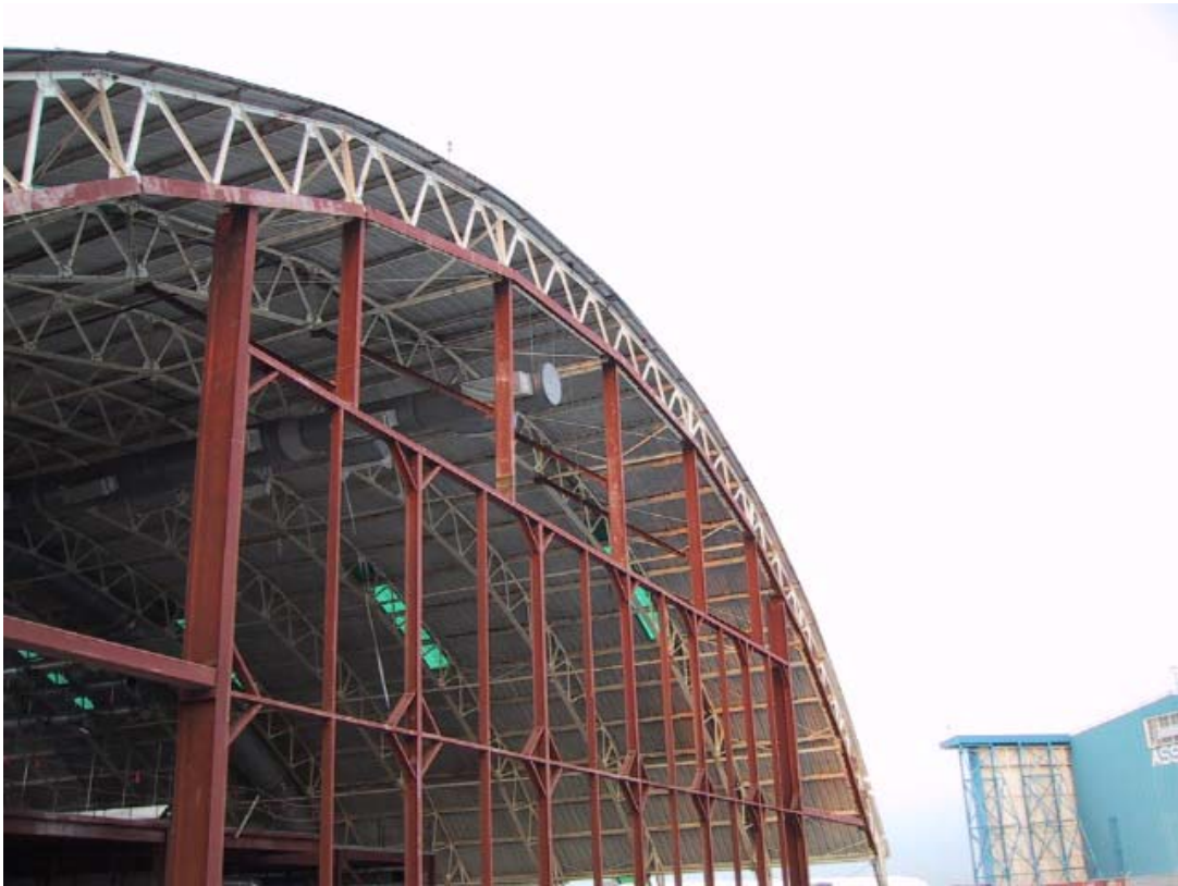
North end of existing hangar being installed
