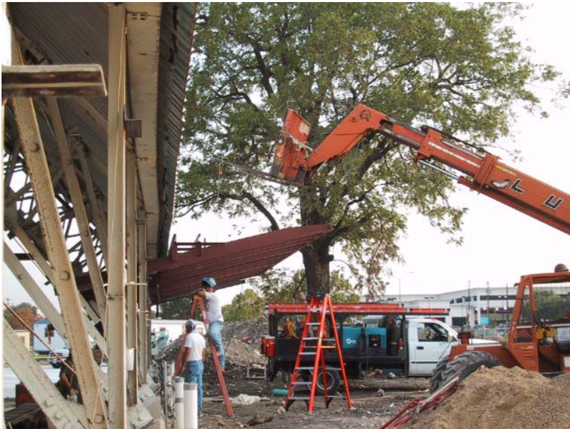
Canopy on Lemmon side of existing hangar going up
