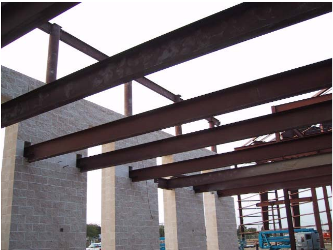
Steel to masonry wall – Gift shop ceiling structure
