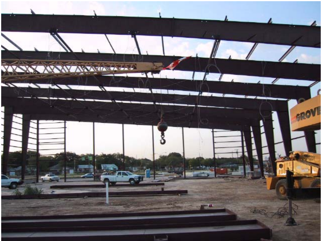
Standing at far North end of hangar looking South – BIG!
