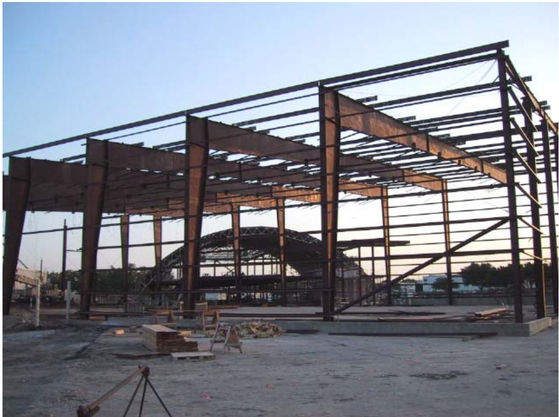
Almost done with pre-engineered building erection
