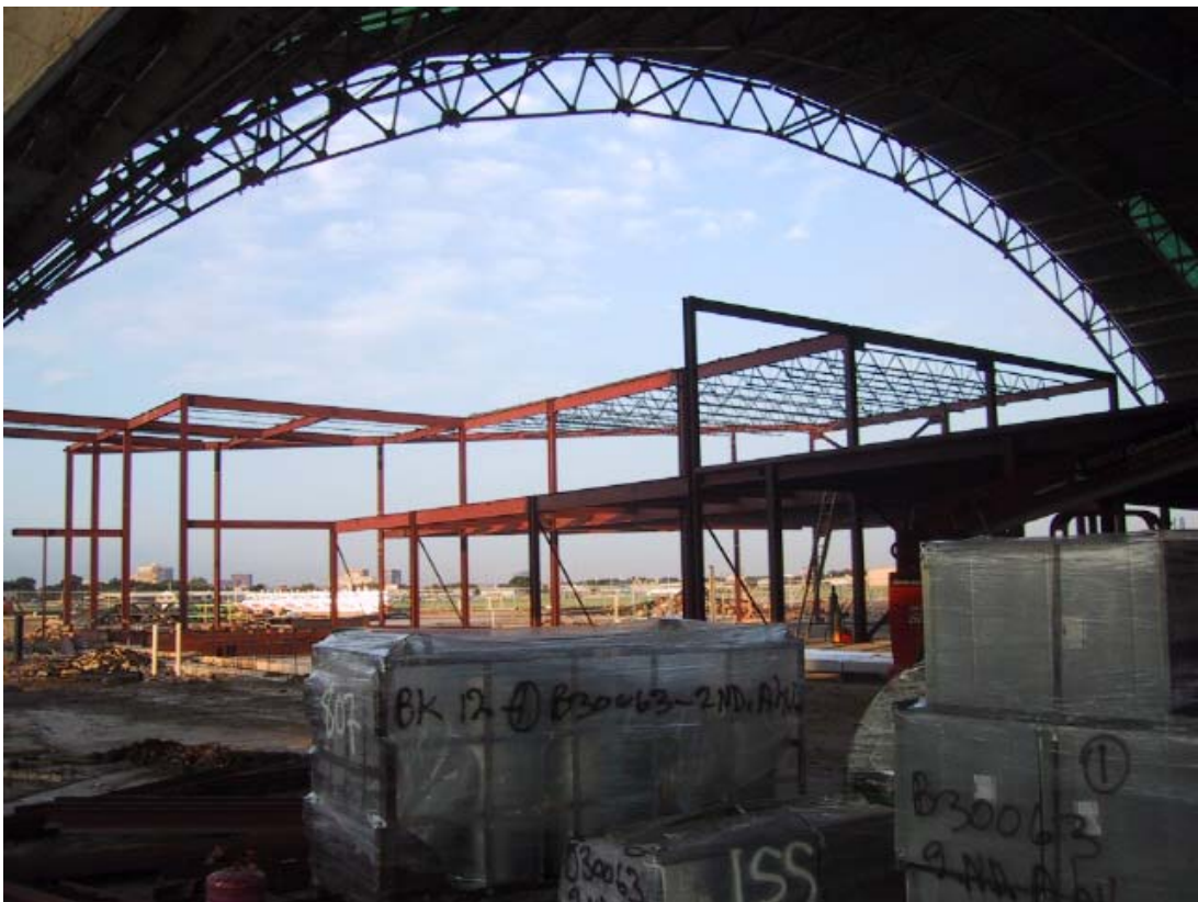
Structure taking shape, ceiling trusses being installed
