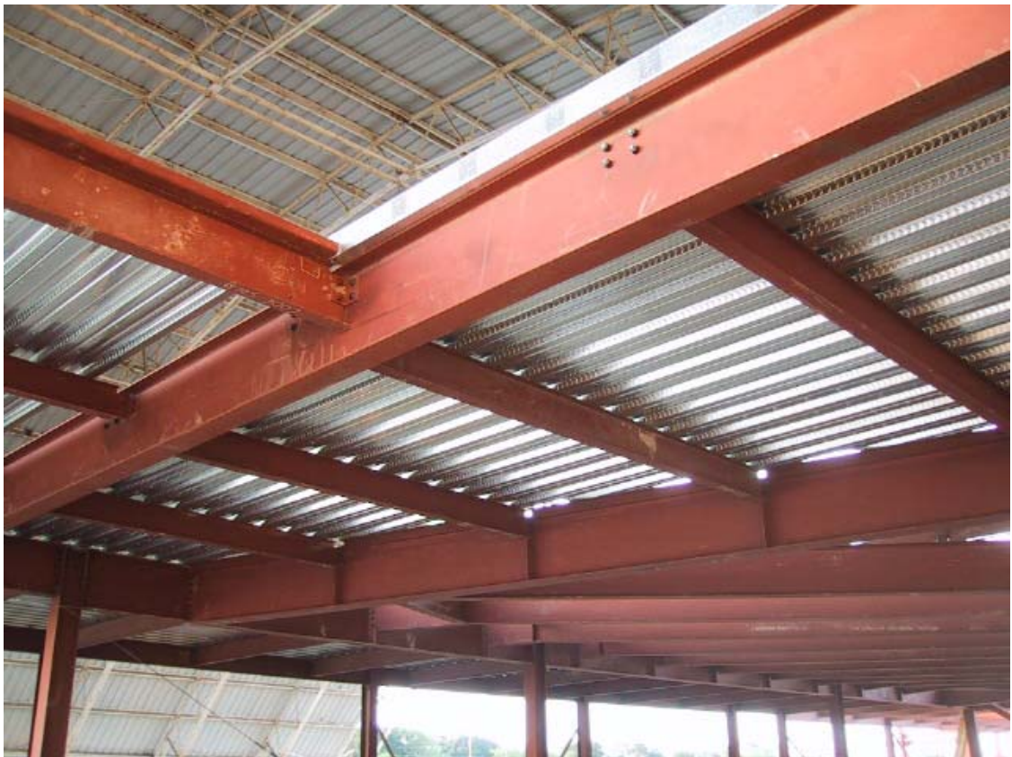
2 nd floor decking being installed
