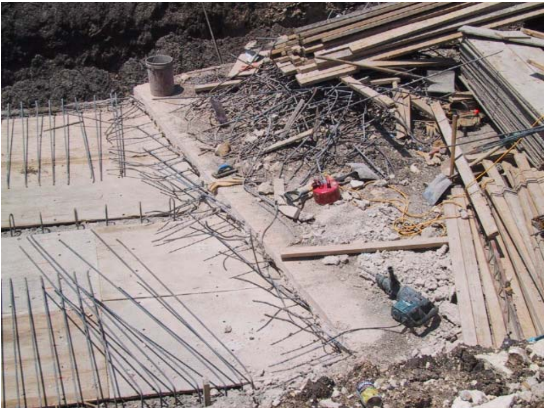
Intersection of new to old culvert at North end
