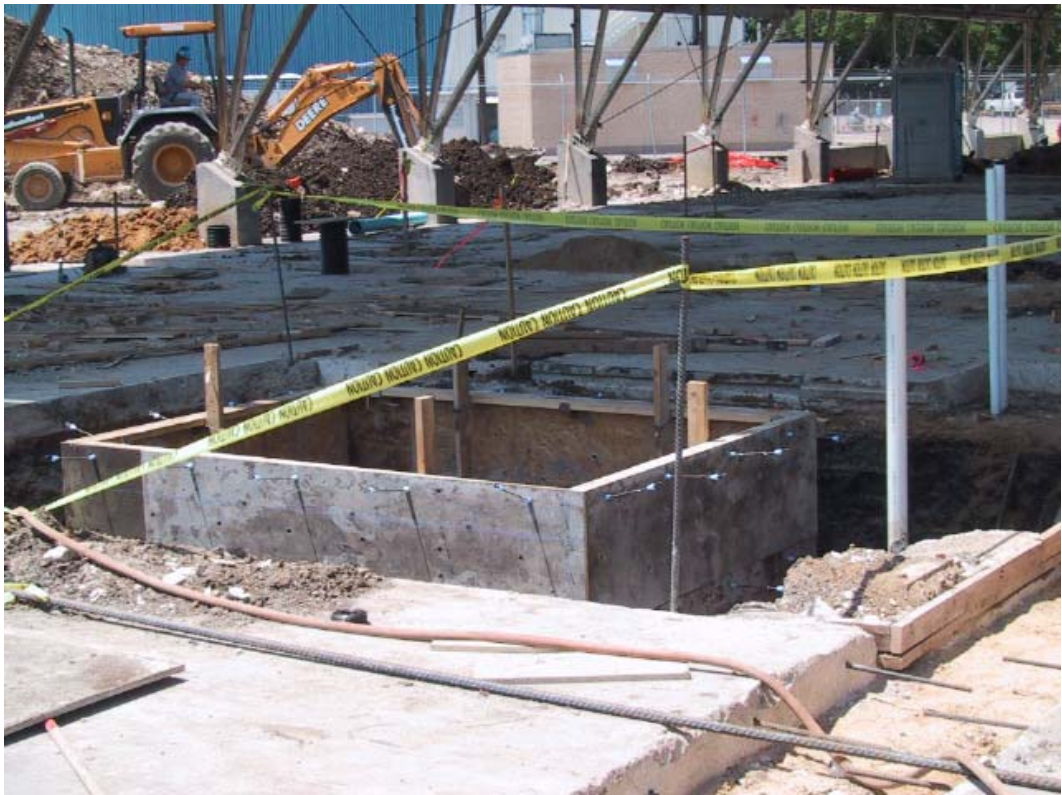
Second elevator shaft being formed (freight elevator)
