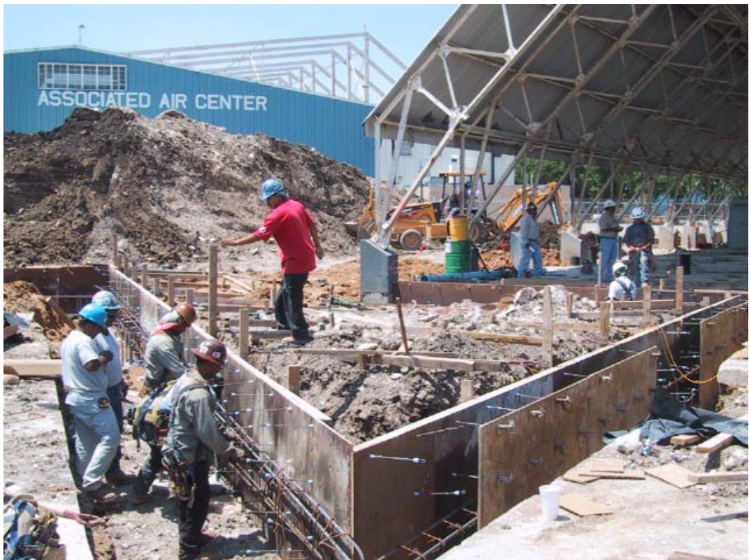
Outline of building nearing completion. Loading dock area shown.
