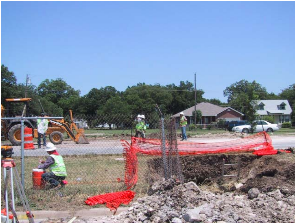
Going under Lemmon for water and sewer
