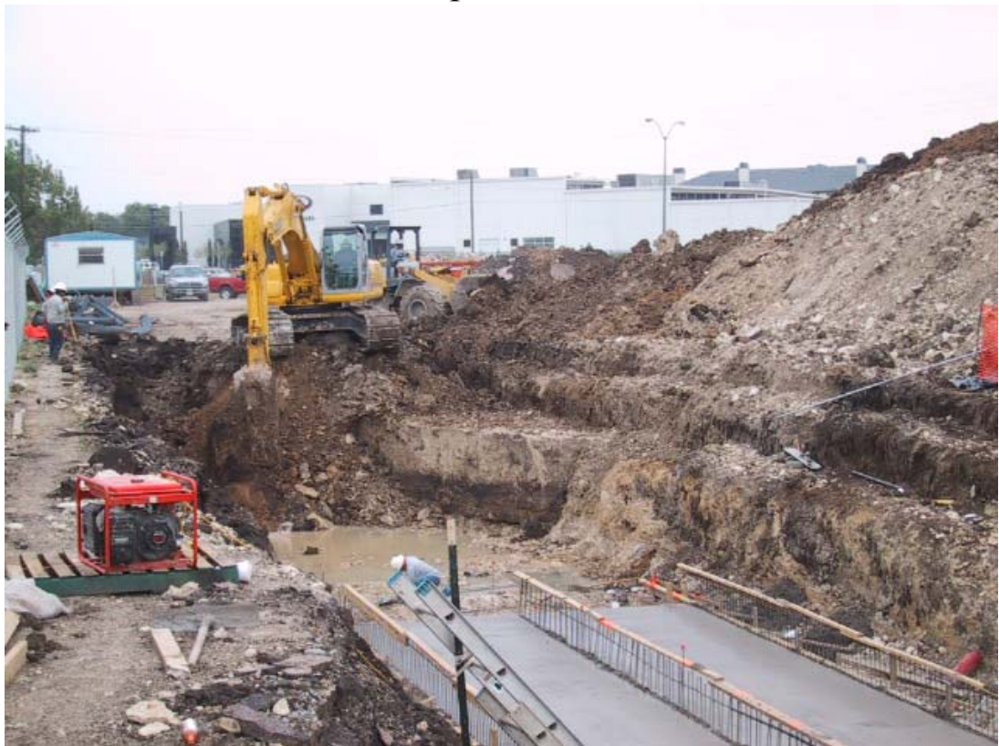
Next step is to tie-in new with old at North end
