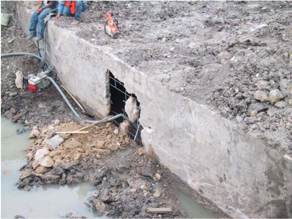
Old culvert reached at South end. Anyone for a little Spelunkering?
