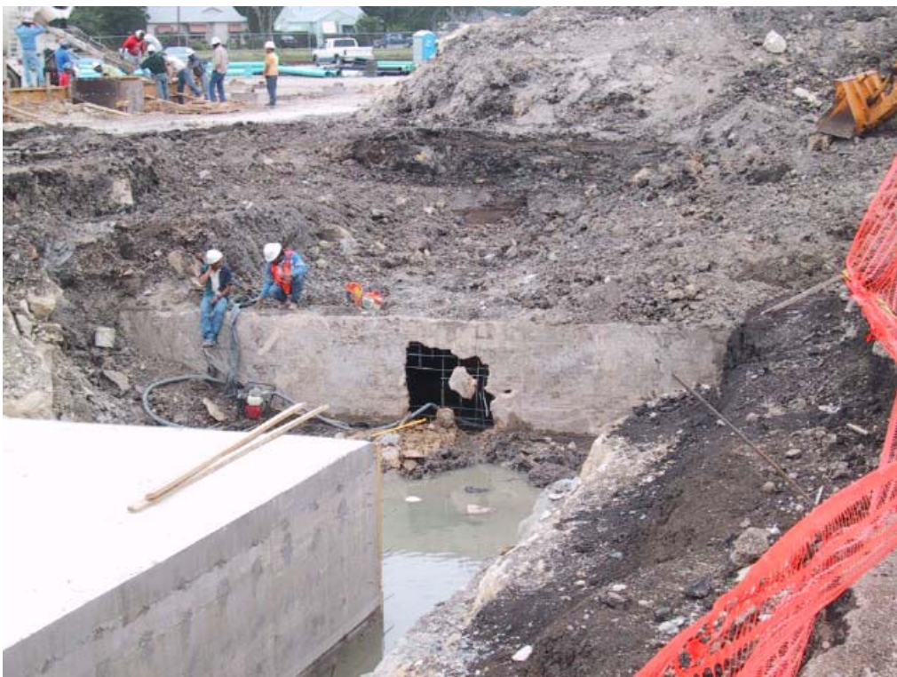
Next step is to tie-in new with old at South end
