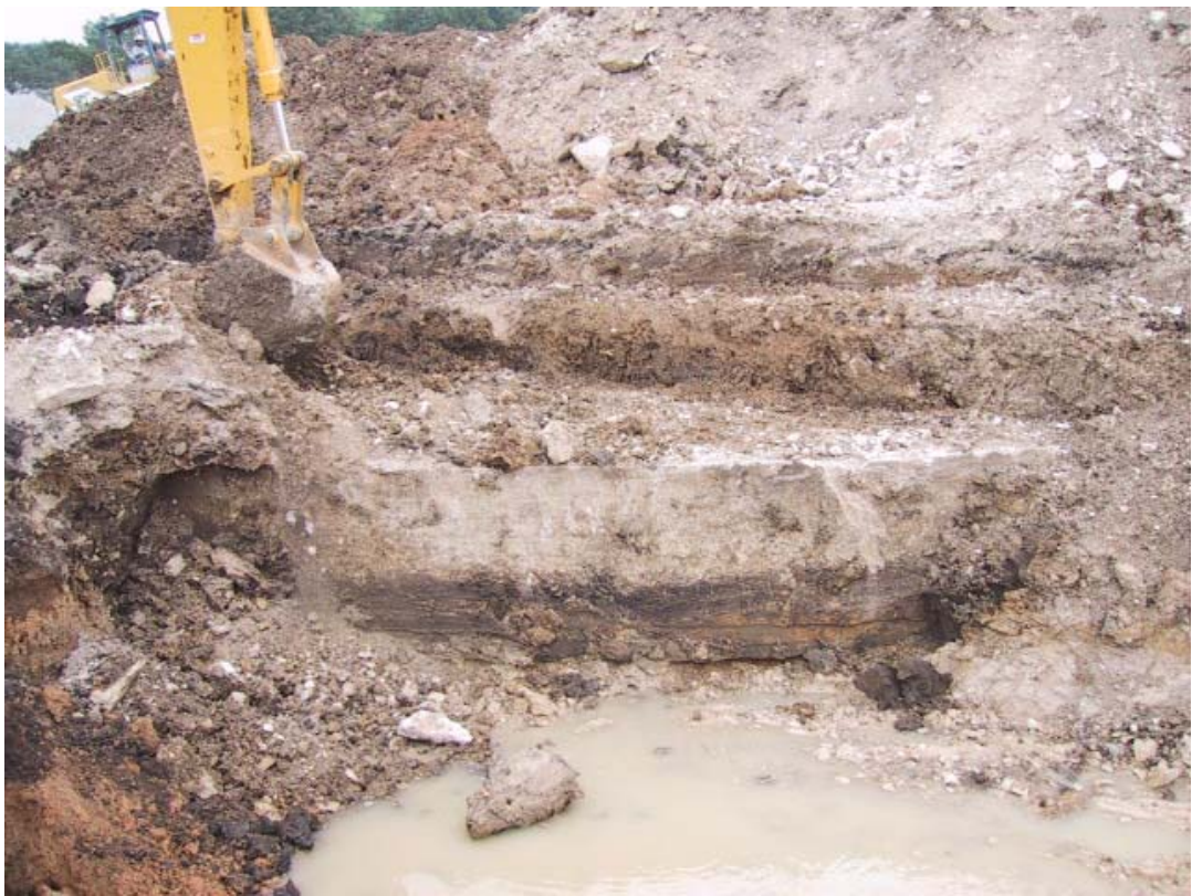
Old culvert exposed at North end
