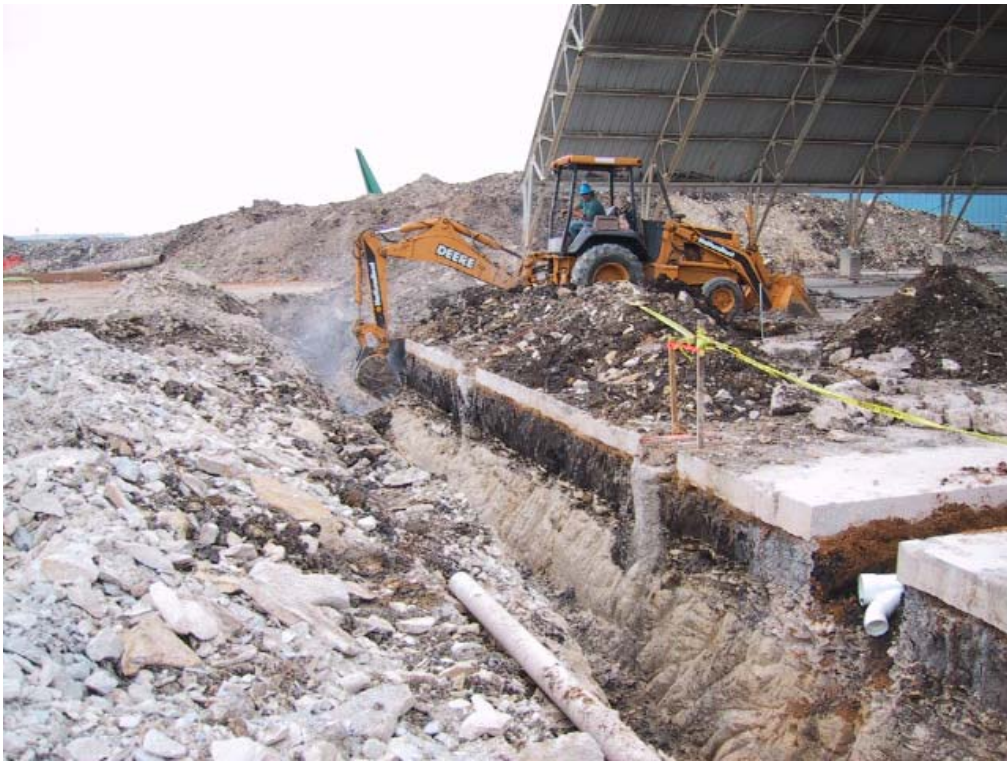
Sewer line trench being dug
