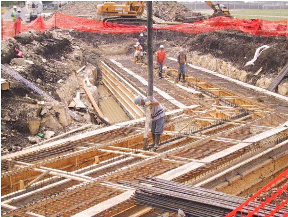
Pouring side walls of culvert
