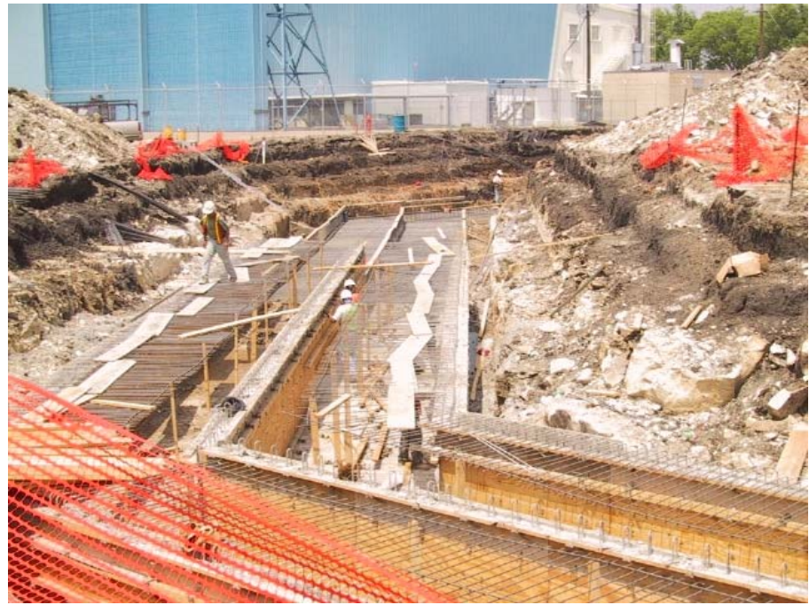
Laying forms for culvert top
