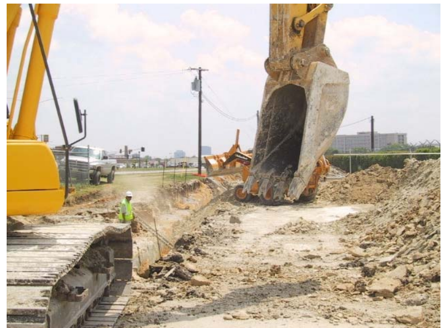
Digging trench along Lemmon to tie into water main
