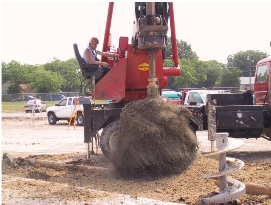
Still digging piers (shaken the dirt off)
