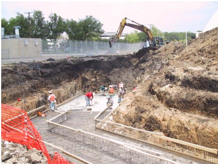
Pouring side walls of culvert
