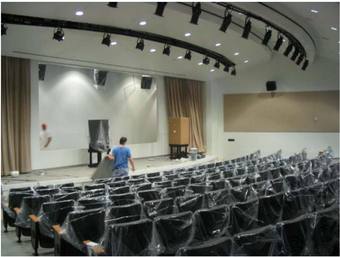
Auditorium seats installed
