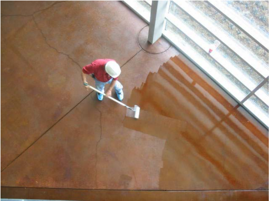
Staining concrete in lobby
