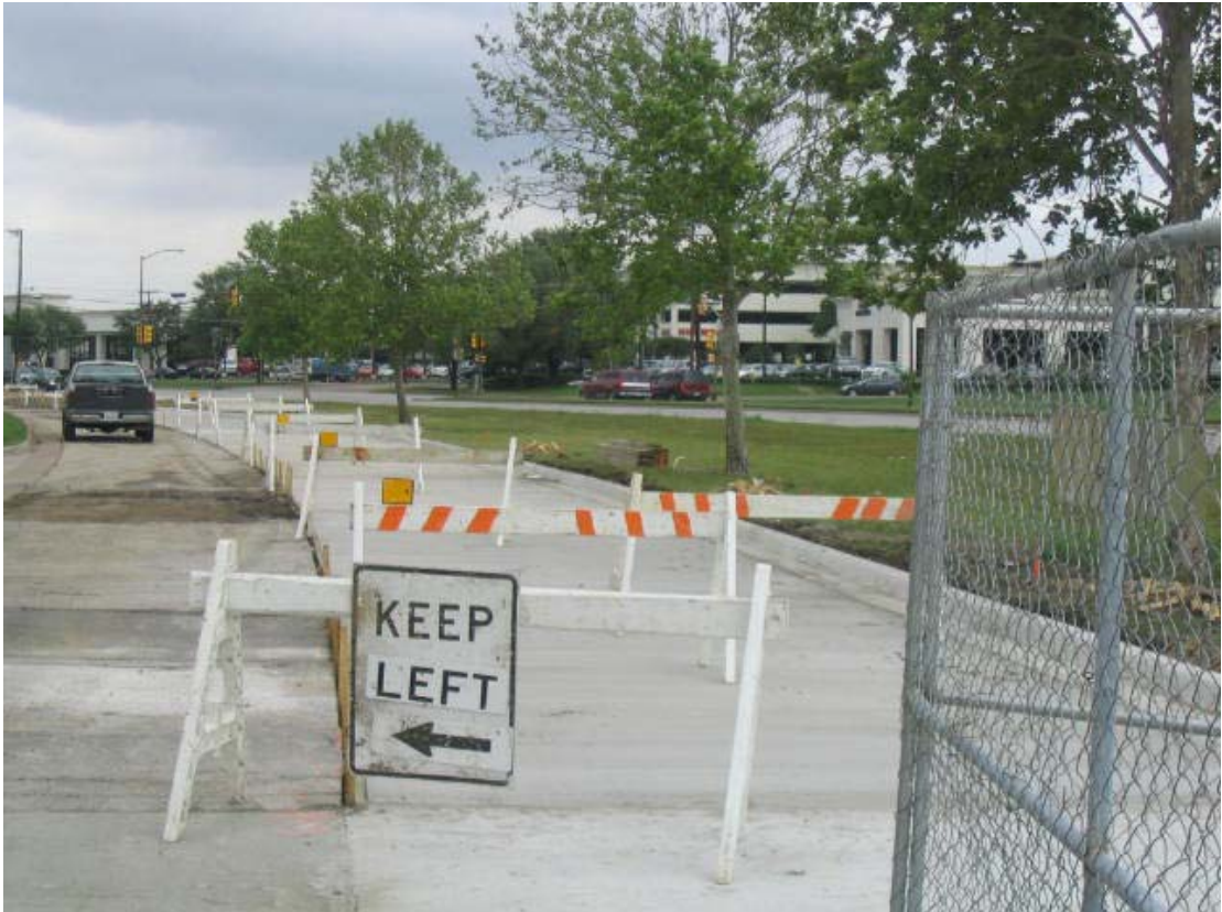
City has started access street widening
