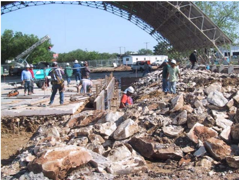
Grade beam work
