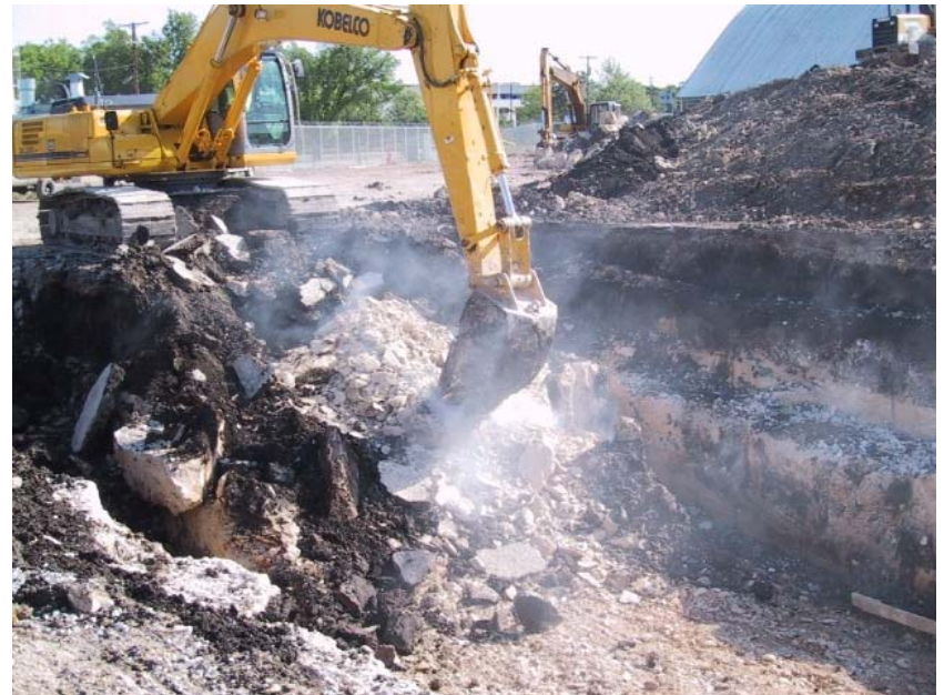
Tough digging for new culvert
