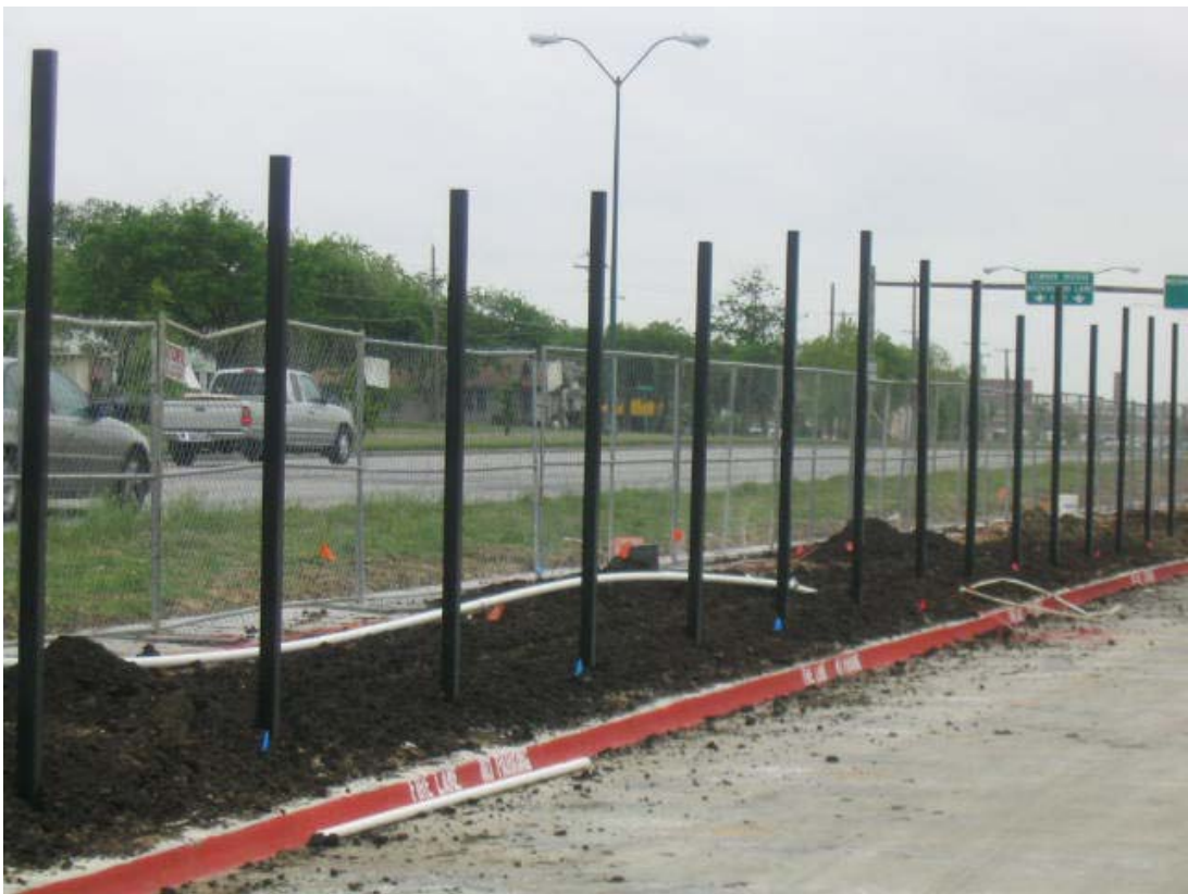
Perimeter fence going up
