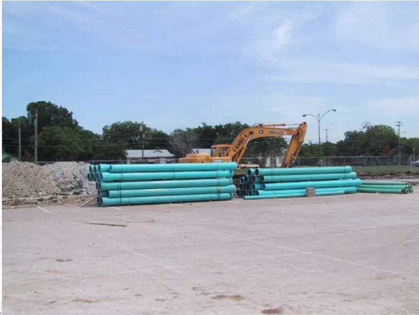
Staged utility piping
