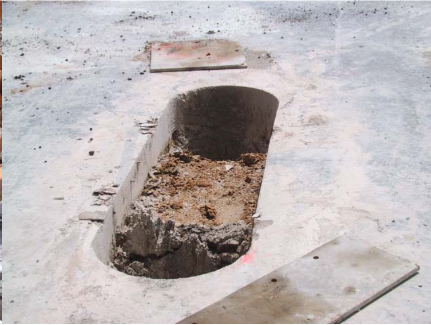
Bridge beam work-around
