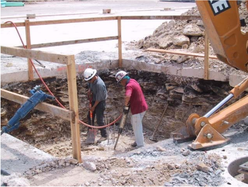
Elevator shaft goes deeper
