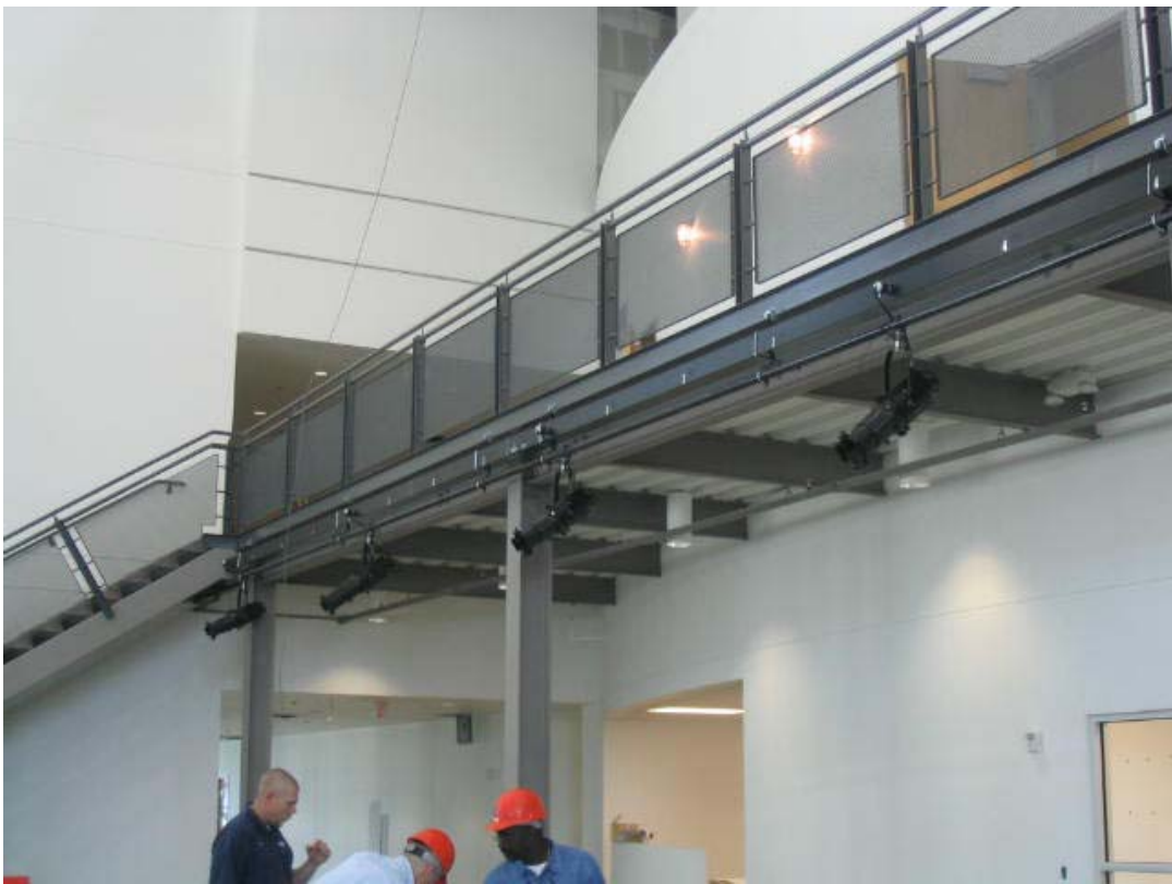
Exhibit track lighting being installed
