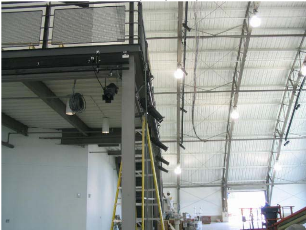
Exhibit track lighting being installed
