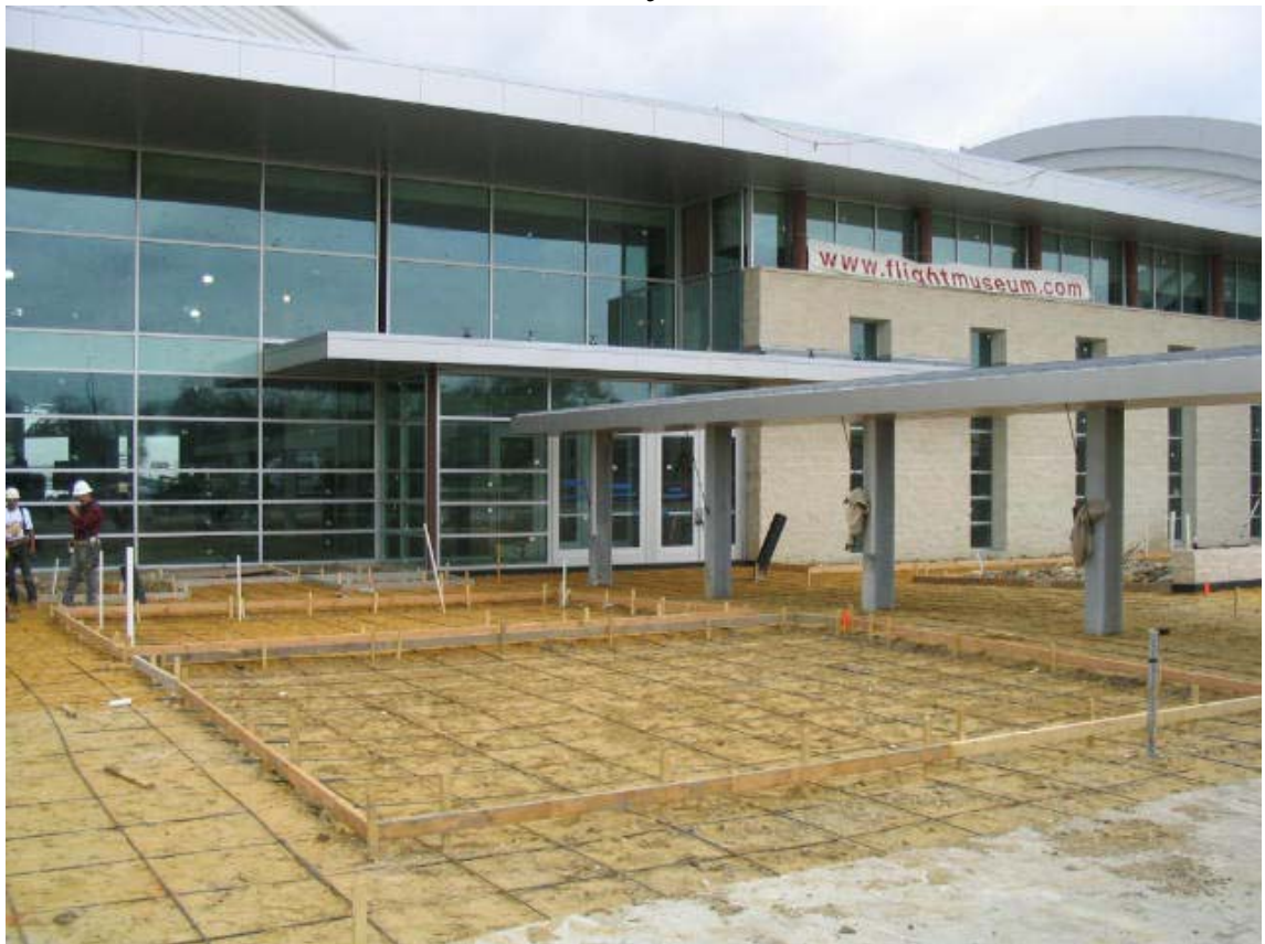
Engraved brick area at entry plaza
