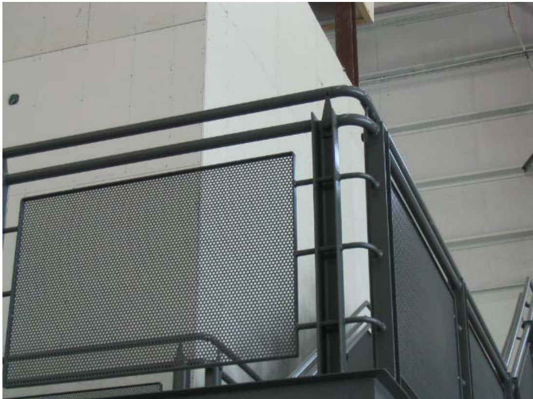
Railing being painted
