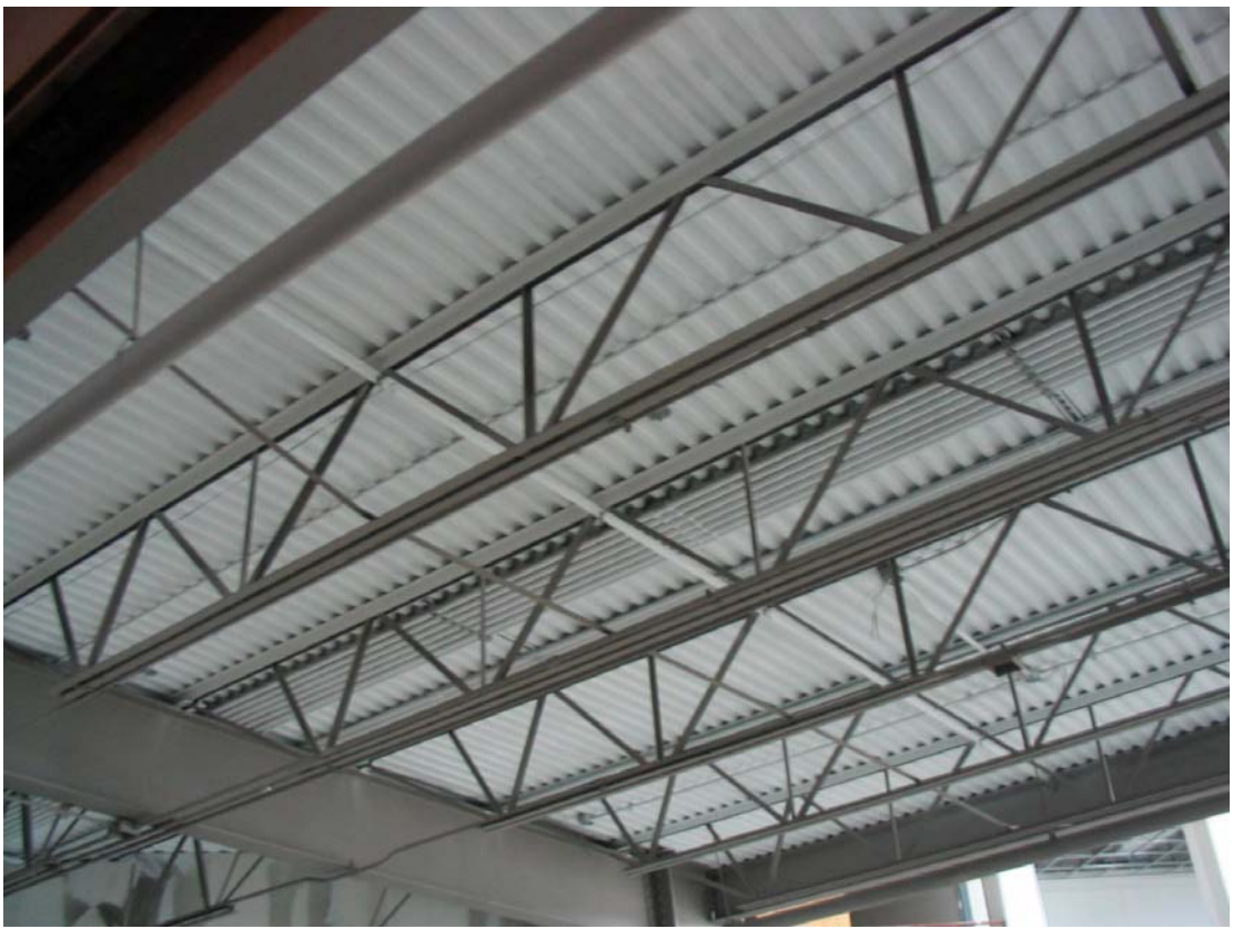
Painting underneath mezzanine deck
