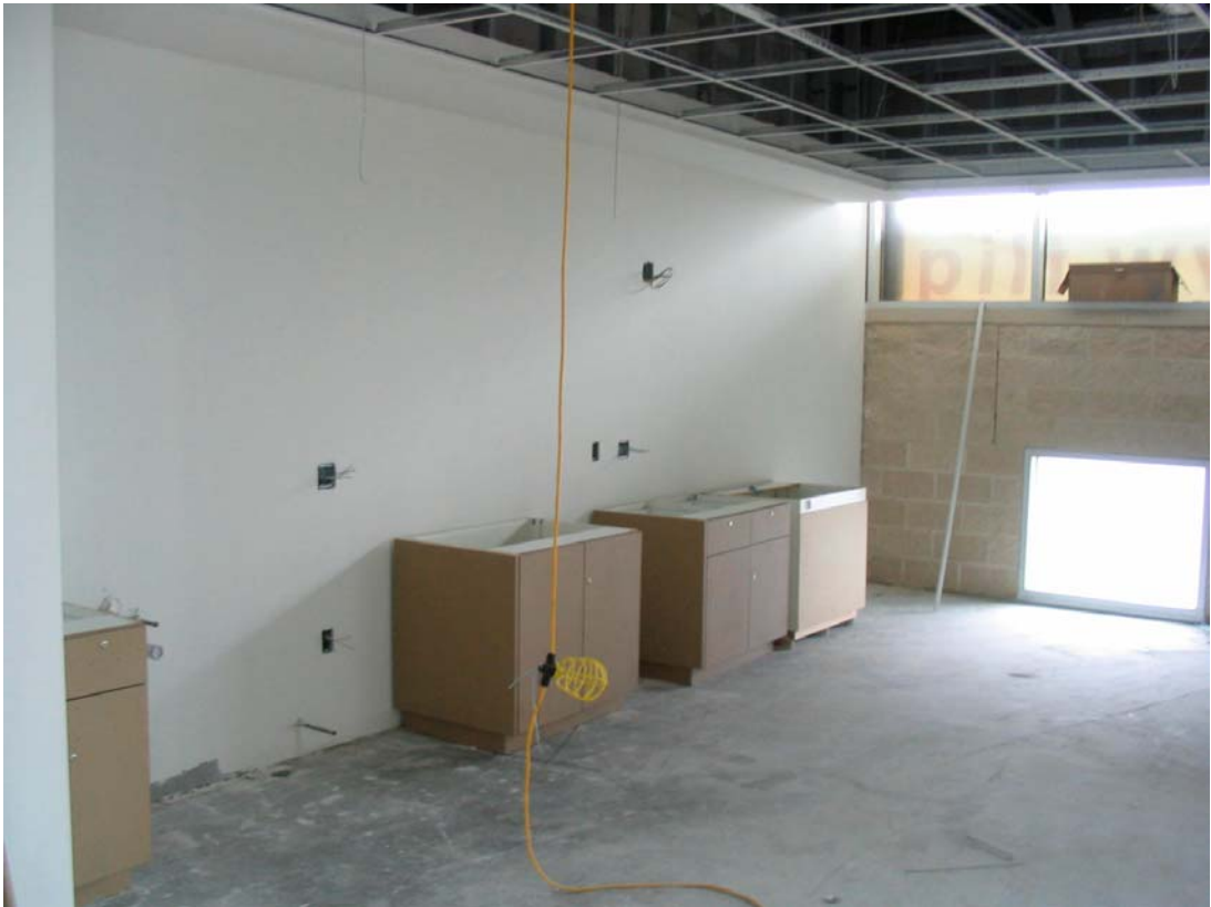
Millwork being installed
