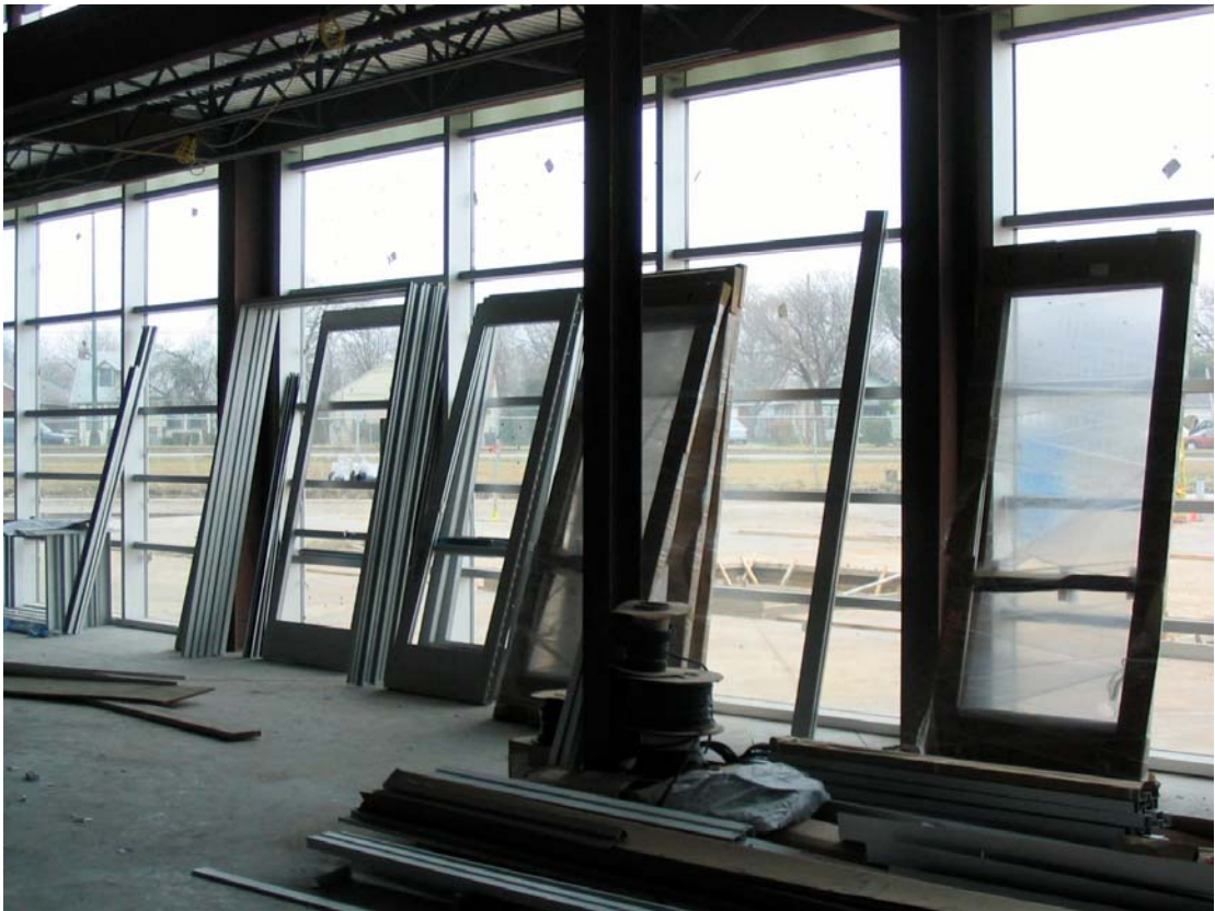
Doors being staged for install
