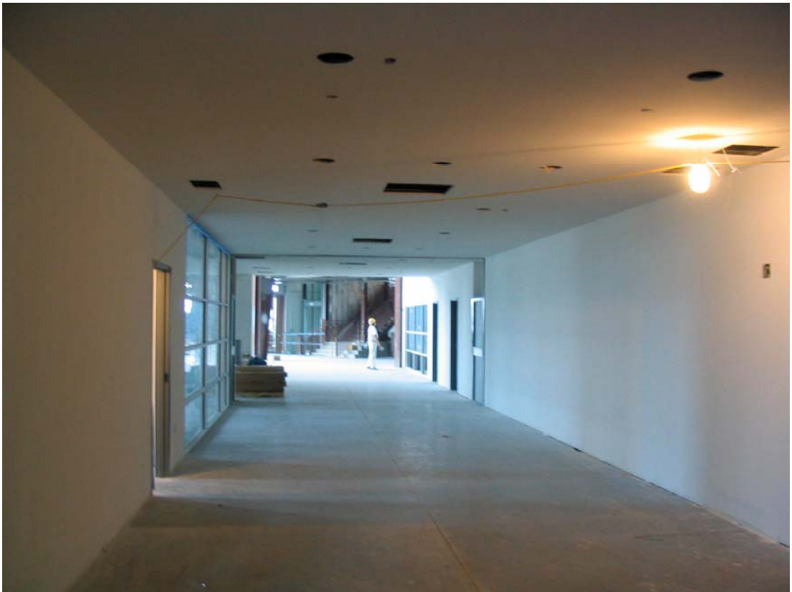
Sheetrock work 90% complete
