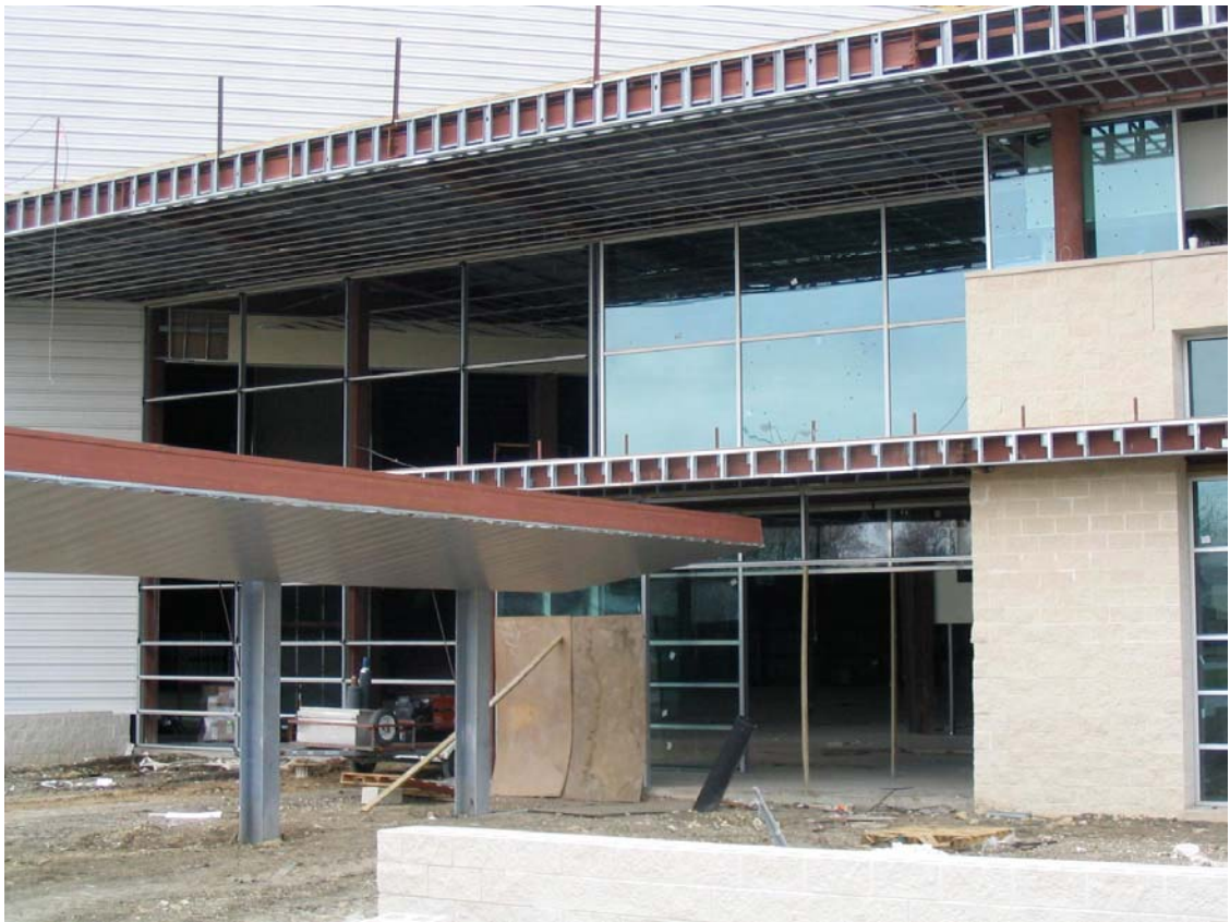
Front entry glass being installed
