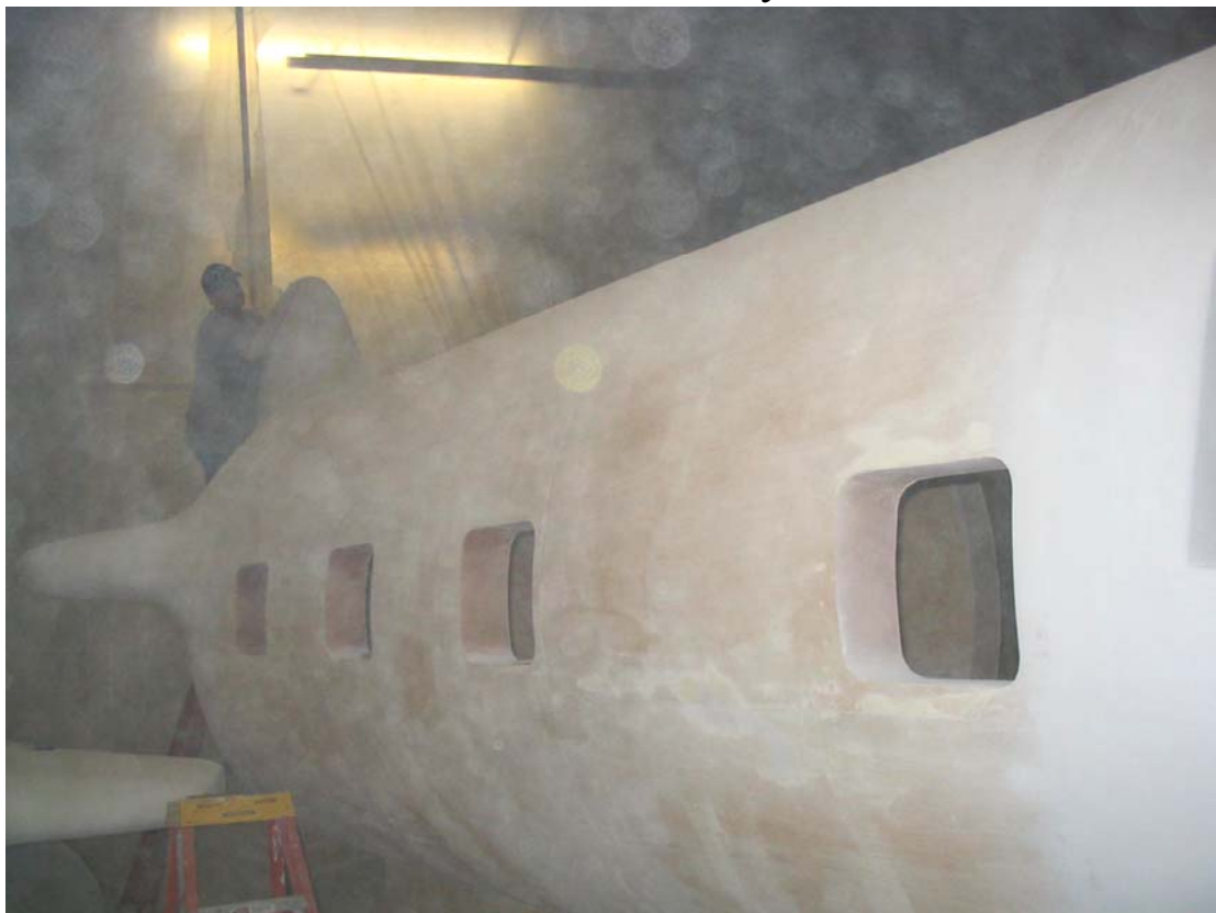
Sneak preview of Kid's education airplane under construction
