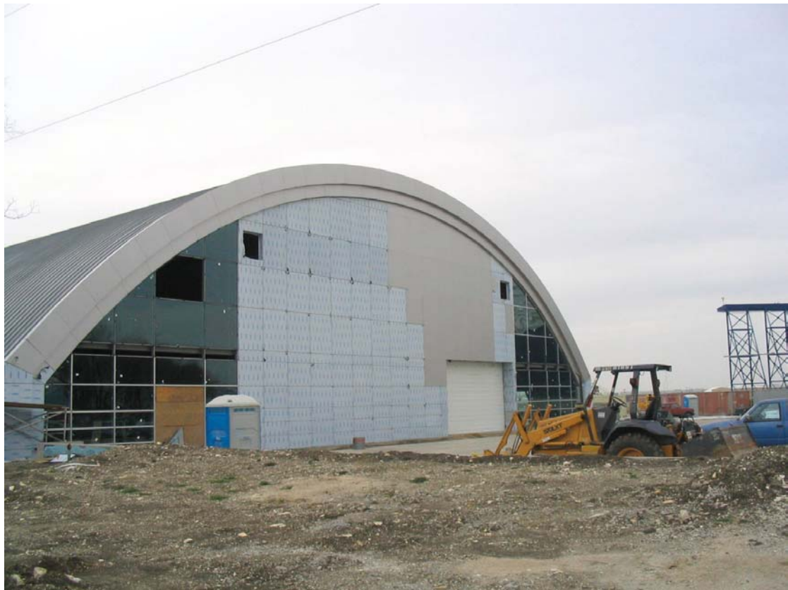
North end Bldg. B - Glass & siding installed
